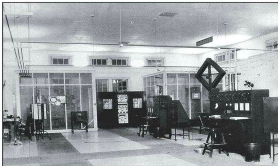
Photo B. Here’s a view inside the Monitoring Room on the north side of the building as it appeared in 1932. This is the same room KDØHKD saw on his tour of the facility in the early 1980s. Equipment included primary and secondary standards and an all-wave receiver. (U.S. Government photograph, courtesy of KDØHKD)
